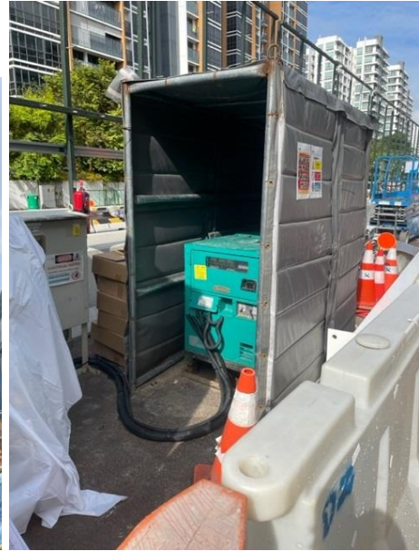
Use of noise shields to house diesel generators
