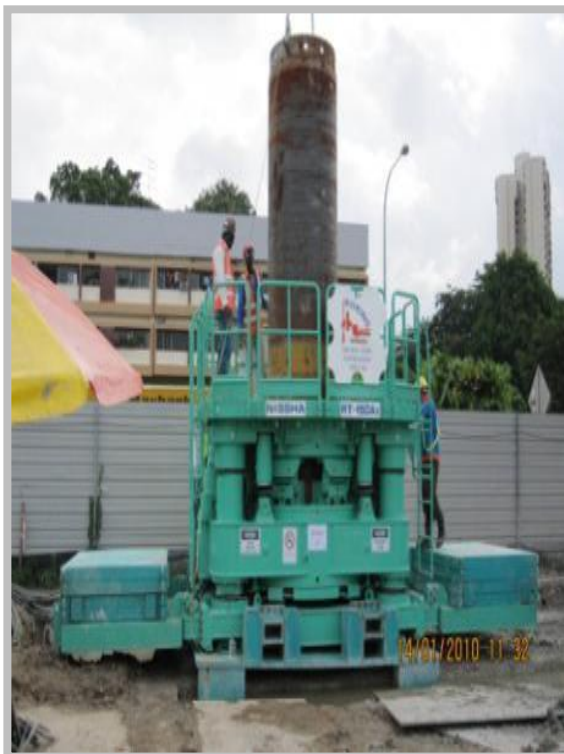
Use of silent-piling machine (for suitable soil conditions)
