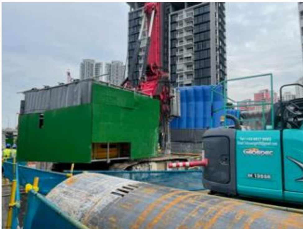
Noise enclosure on boring rigs
