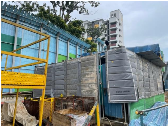
Use of noise shields to house diesel generators
