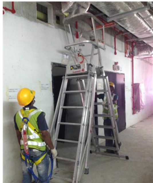
Examples of Step Platforms being used on site
