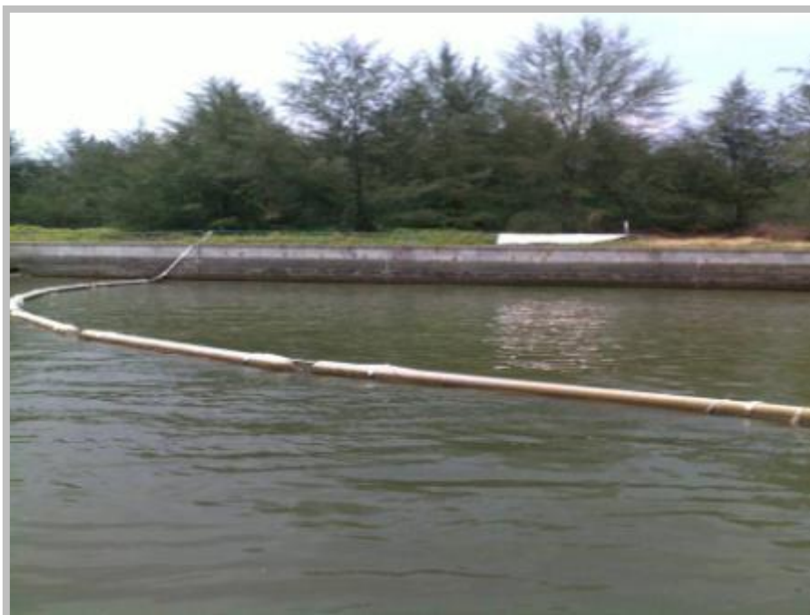
Adequate use of turbidity curtain for works near water-bodies / waterways
