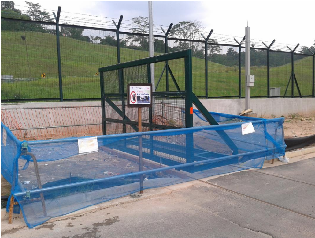
Cordon off work zone around gate installation
