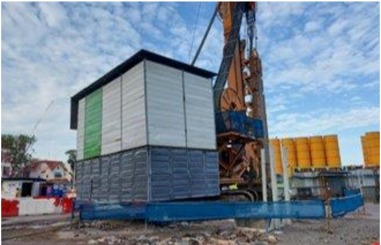
Use of localised noise barriers for noisy machinery (eg. Diaphragm Wall Cutter)
