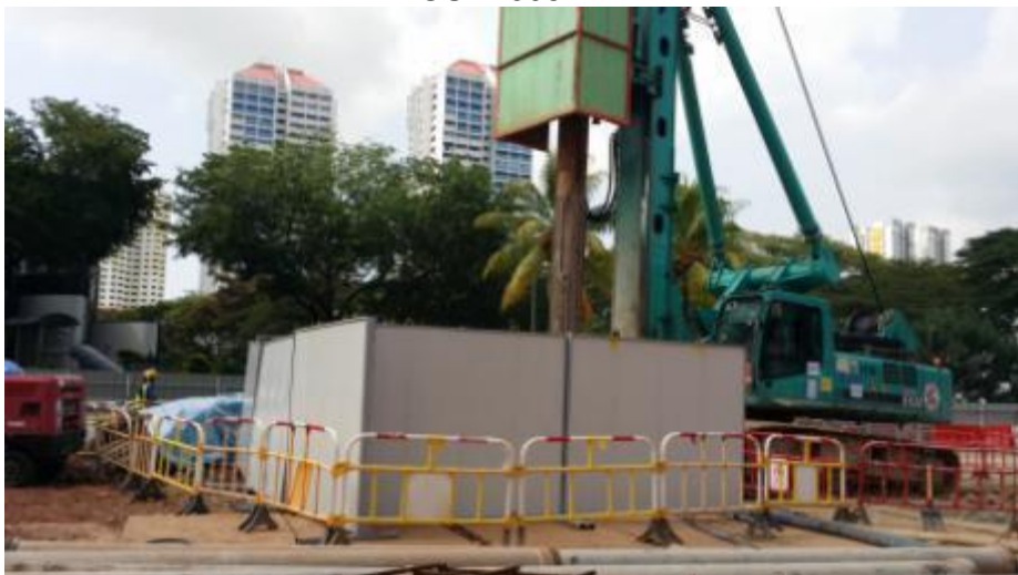
Use of portable noise barriers around noisy works such as bore piling
