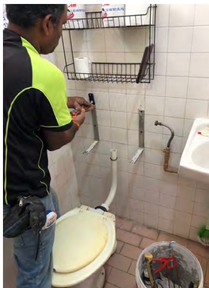
Pro-bono contractors from Ideal Plumbing Pte Ltd assisting to replace toilet cistern set.
