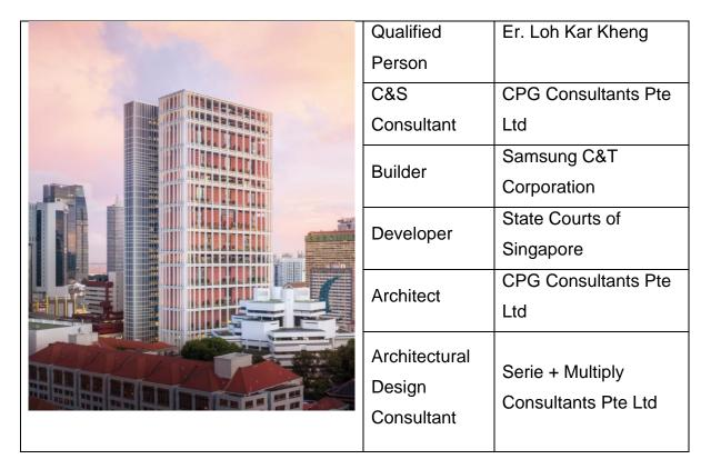
The new 35-storey State Courts Towers comprises two towers, the 'Court Tower" and a very slender "Office Tower". At 178 metres high, it is the tallest government building in Singapore to date. The Court Tower has an open frame building facade, with courtrooms stacked on each other, resulting in aesthetically pleasing slender Court Tower Columns, consisting of long span floor slabs/beams and columns sizes befitting the facade.
