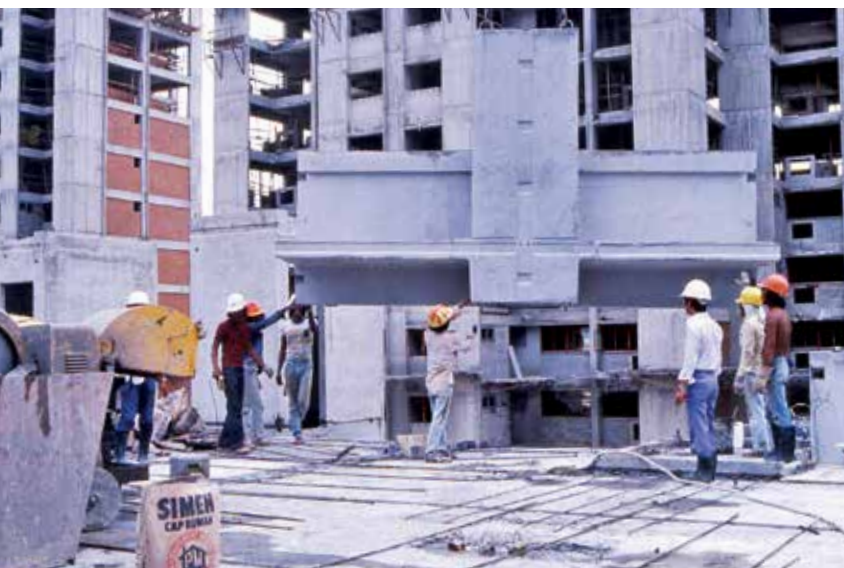
Builders using prefabrication technology in the construction process.
